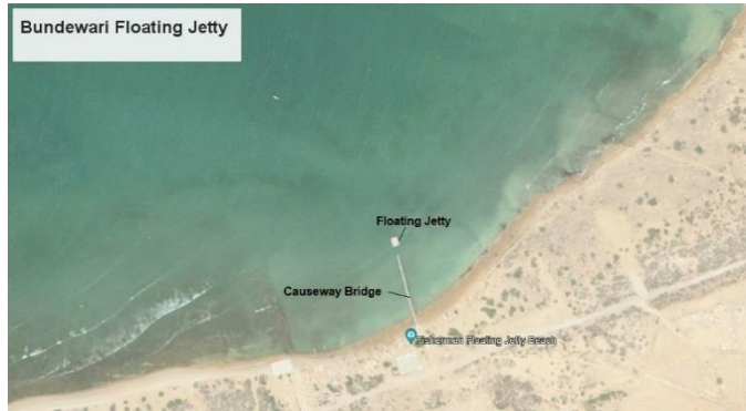
Fig. 7. Floating jetty at Bundewari (Lasbela)
